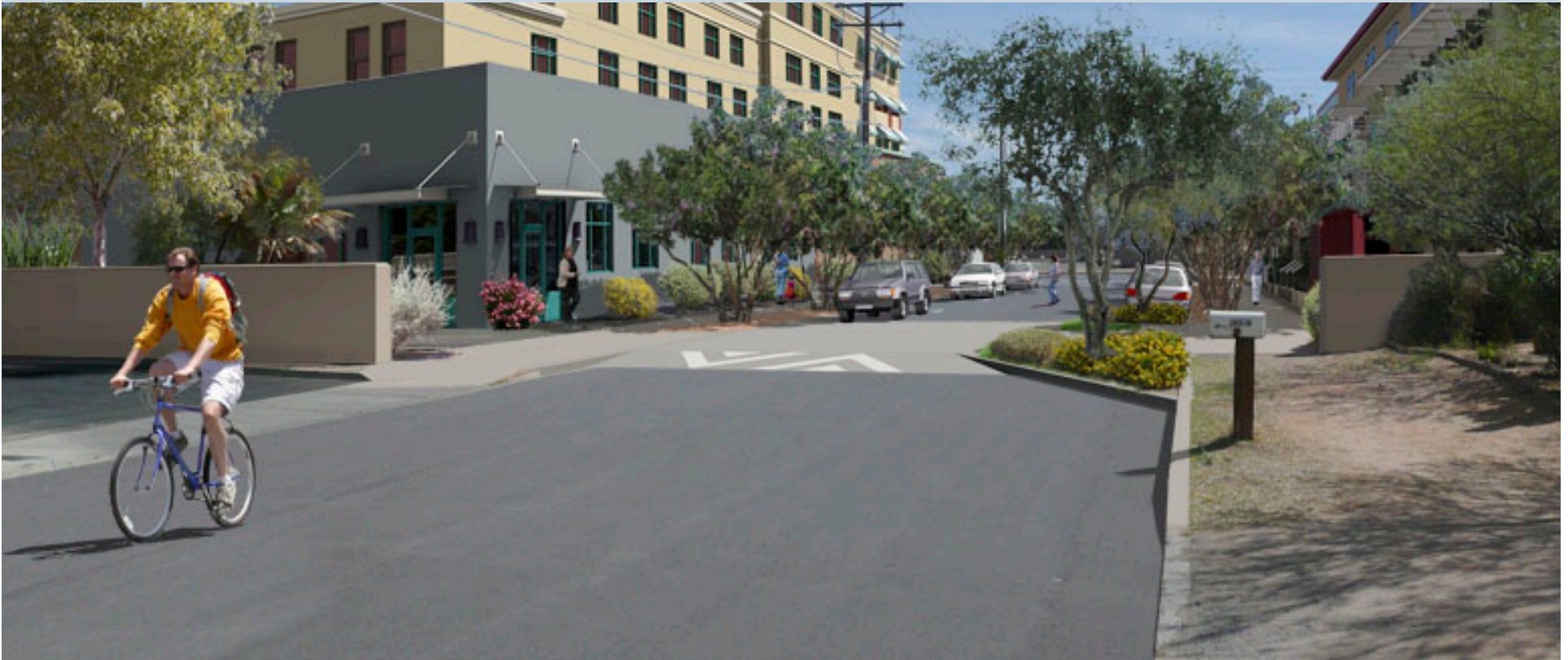
Example Chicane and Speed Table
