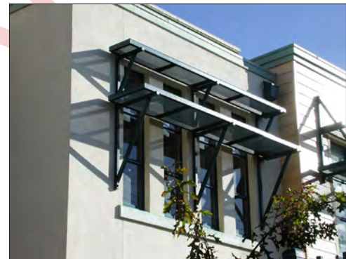
Figure 5.10.2.d and 5.10.2.e: Photo examples of shading devices that integrate with building and site design; the shading device on the left is to provide shade for pedestrians passing along the edge of a plaza and the device on the right provides shade and building articulation.
