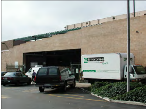
Figure 5.7.5.a: Photo example of loading facilities within the building envelope.
