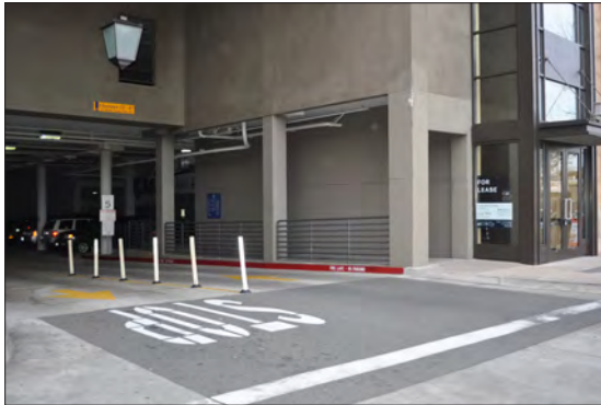
Figure 5.7.1.f: Photo example of a driveway entry that accommodates pedestrians with a walkway.
