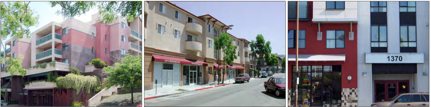
Figure 5.6.2.k through 5.6.2.m: Photo examples of building articulation. Figure 5.6.2.k above does not meet the articulation standards because it relies on color changes without changes in mass or materials while the building in Figure 5.6.2.l does not have enough articulation of the upper facade. Figure 5.6.2.m is an example of a building that satisfies the articulation standards with a combination of massing, materials, and color.
