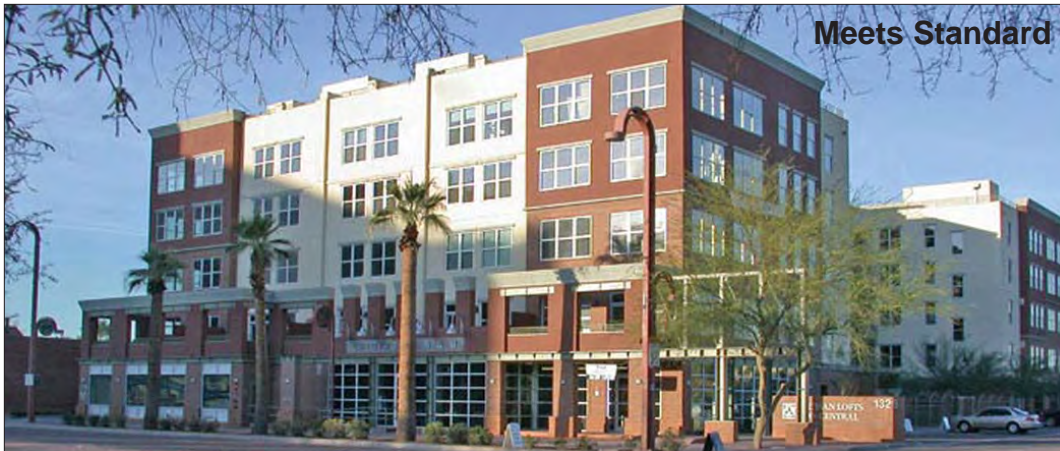
Figure 5.6.2.b: Photo of example building that meets the standard for massing with a logical rhythm and order, where the massing articulation relates to the rooms within the building, and frames both ends of the building.
