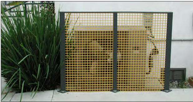
Figure 5.7.5.d: Photo example of an exterior utility screen designed to complement the architectural design of the building.
