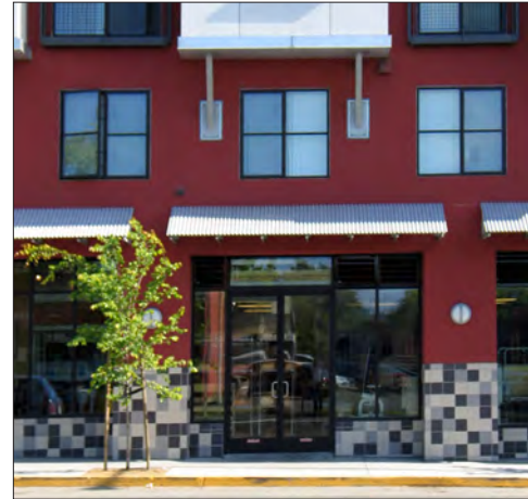
Figure 5.6.2.r: Photo example of a main entrances that has composition and articulation that make it human-scaled.
