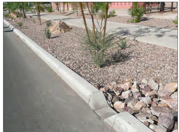
Figures 5.4.4.cc and 5.4.4.dd: Photo examples of passive water harvesting associated with street improvements in Tucson.
