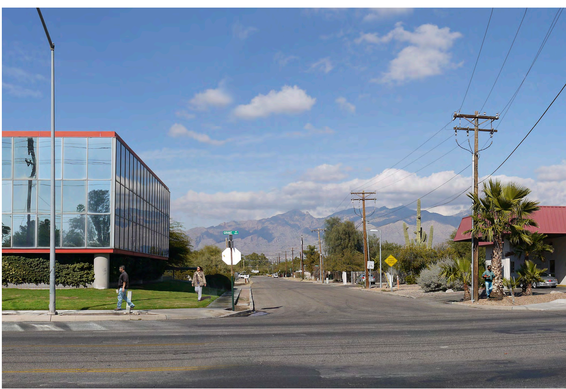
Grant Road is an important east-west connection for people throughout the Tucson region.
