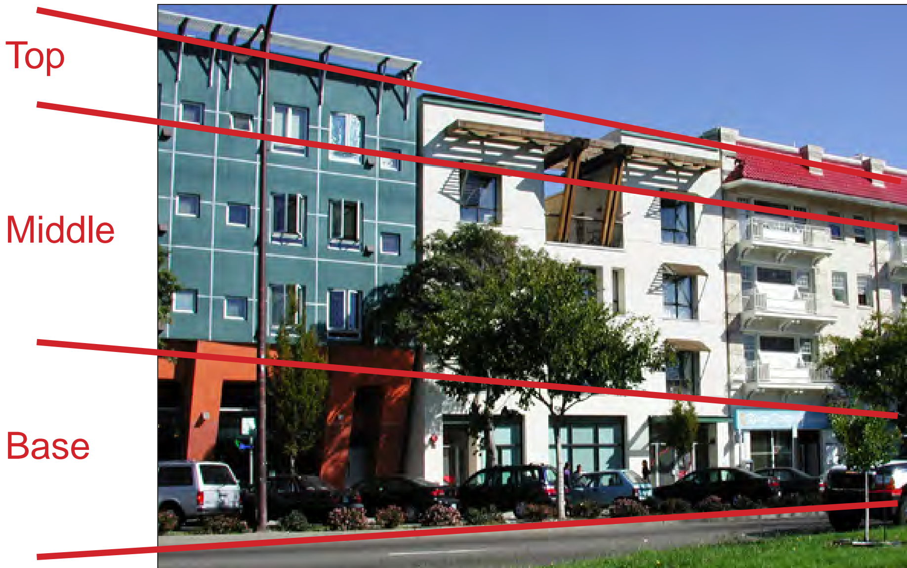
Buildings must be composed of a base and top that are human-scaled.
