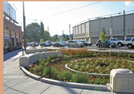
Passive water harvesting in median, similar to side median in 160' right-of-way.
