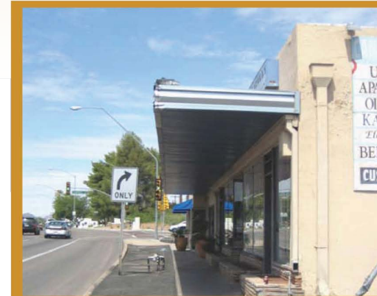
Existing storefront at Campbell and Grant
