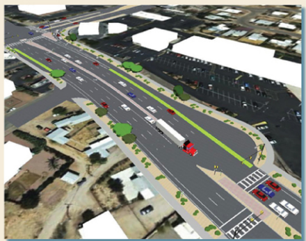
The 'bulb out' allows U-turns for larger vehicles such as buses and semi-trucks.
