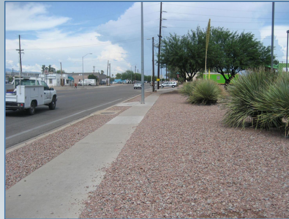
Landscape outside of sidewalk
