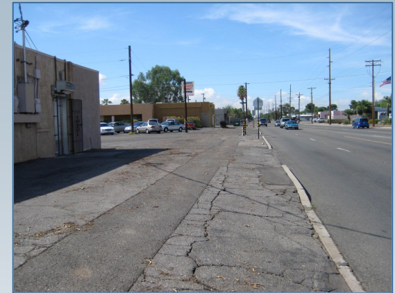
Frequent curb cuts
