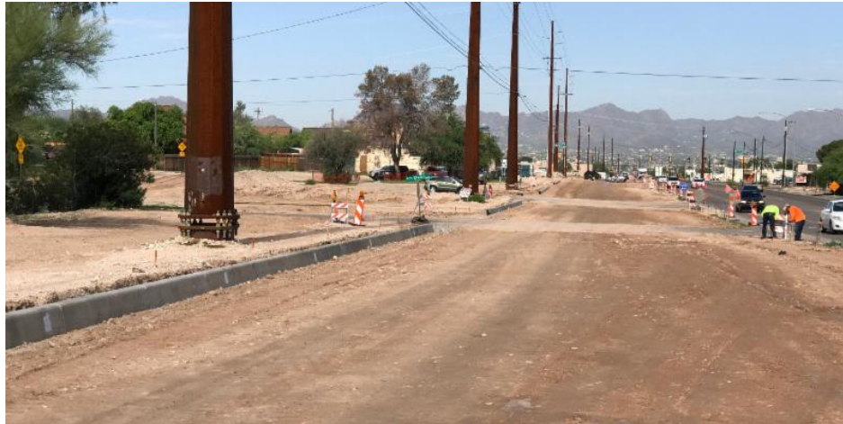
New curb installed on July 26, 2017
